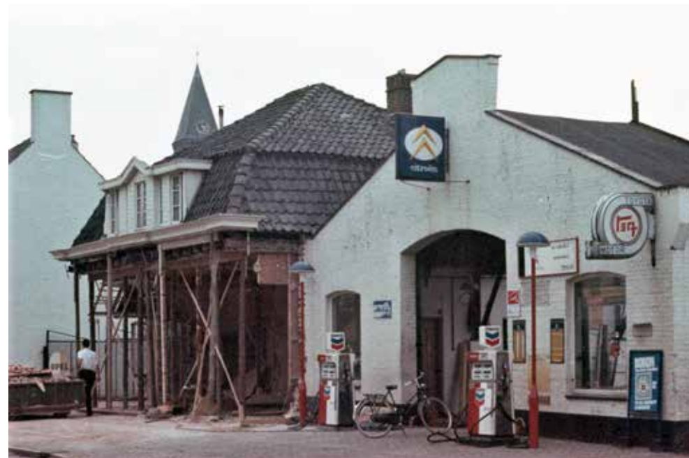
De verbouwing is in volle gang, 1970.
